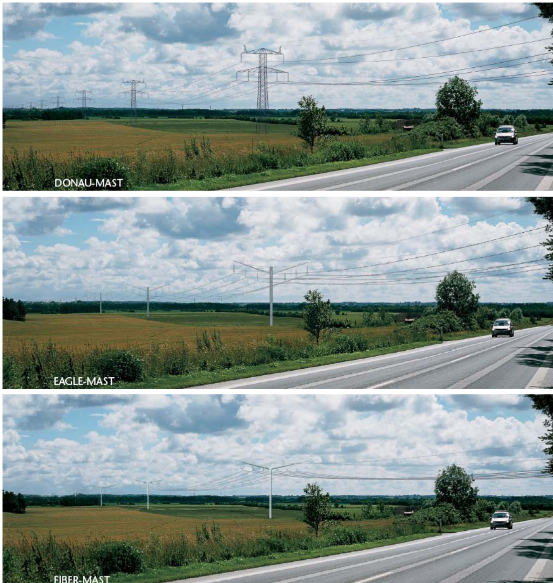
Figure 7 Existing and new tower types – all intended for two 400 kV systems. The Danube tower is used in several places in Jutland. The development of the Eagle tower has been completed, and the tower can now be used in new projects. The fibre mast is currently being developed and will presumably be ready for use in approximately five years.
